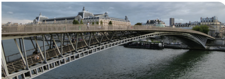
The Paris Soferino Bridge's walkway is made of Ipe wood.
